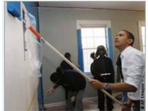
Barack Obama takes part in a renovation of a homeless shelter for runaway teenagers in Washington on January 19.
